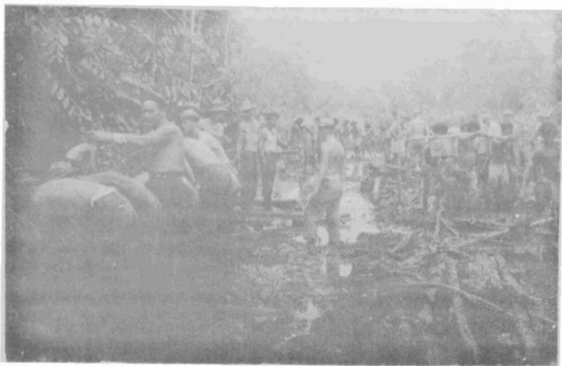
Building jeep-track from Sinemi Village to bridge between the strips. . .
